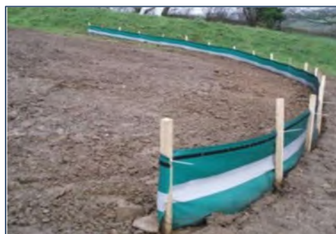
Plate 4-6. Embedded Silt Fence
