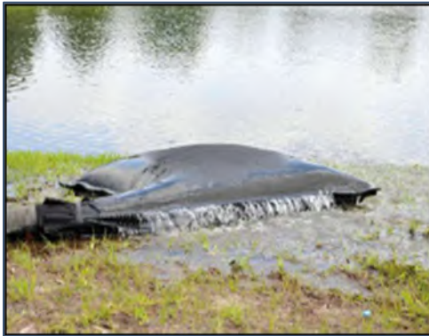
Plate 4-3. Silt Bag with water being pumped through.
