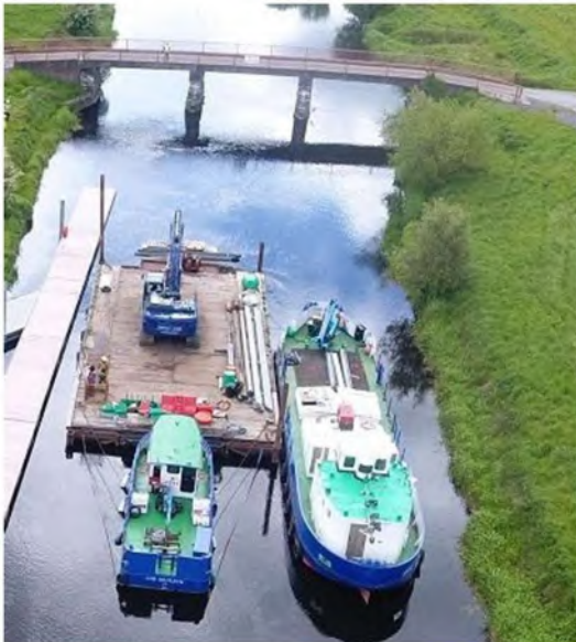
Plate 4-2 Coill an Eo, Inis Muilinn workboats and Pontoon Raft with 36-tonne excavator
