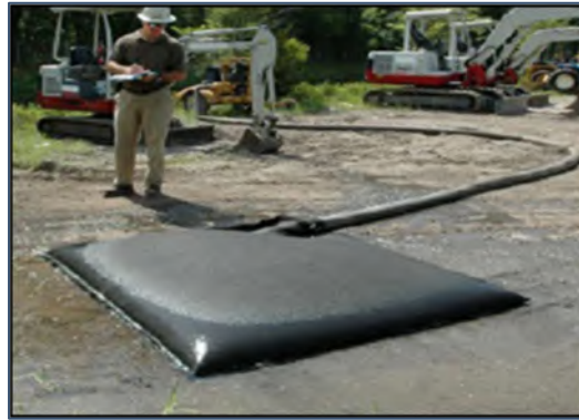
Plate 4-4. Silt Bag under inspection.
